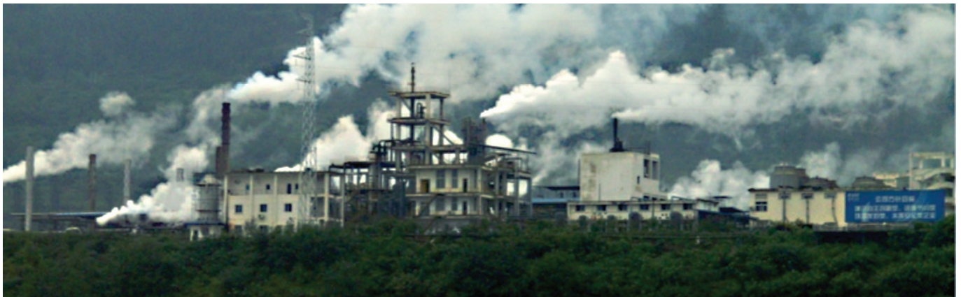
Factory on the Yangtze River, China, 2008. Photo by High Contrast (Permission under CC BY 2.0).
