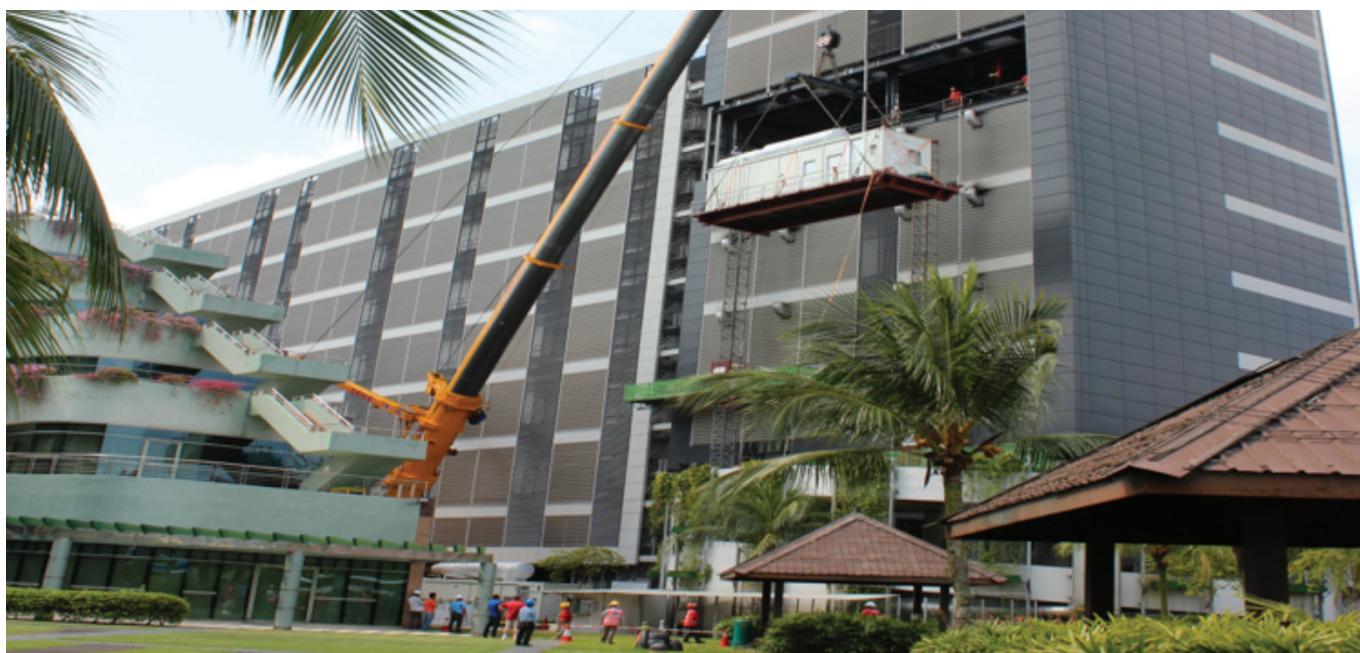
Air Conditioning Equipment Installation in Singapore, 2012. Photo by RudolfSimon (Permission under CC BY-SA 3.0).
