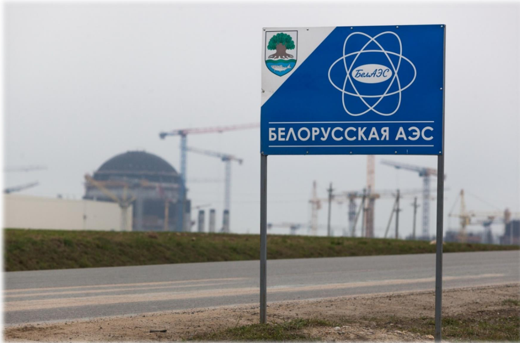
Belarusian NPP under construction
