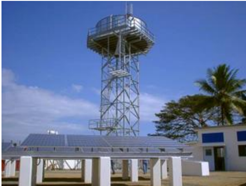
Rural water supply facility using solar energy in Papua New Guinea. www.jat.co.jp/english/services/sv3/
