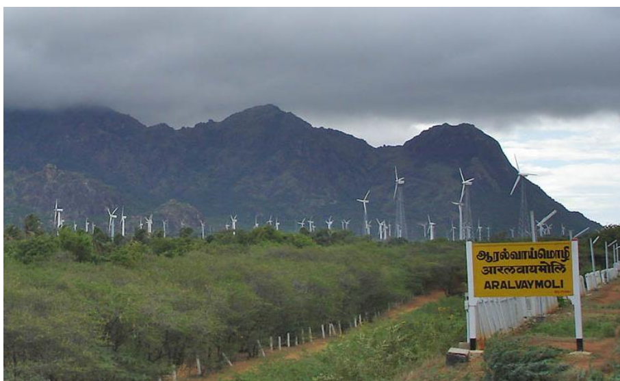
Aralvaimozhy railway station with a view of Muppandal wind farm Permission under CC BY-SA 2.5 commons.wikimedia.org/wiki/File:Aralvaimozhy_station.jpg
