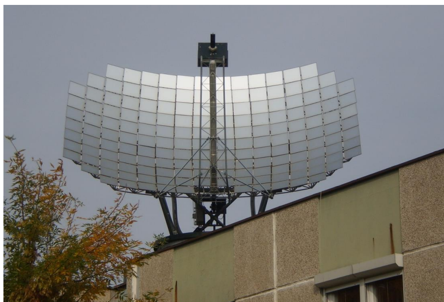
Solar parabolic array of mirrors for domestic water heating by Kaboldy. Permission Under CC BY-SA 3.0 commons.wikimedia.org/wiki/File:Solar_parabola.jpg
