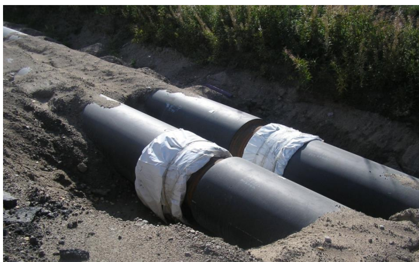
District heating pipes in Jyväskylä by Antti Leppänen. Permission Under CC BY-SA 3.0 License commons.wikimedia.org/wiki/File:District_heating_pipes_in_Jyv%C3%A4skyl%C3%A4.jpg
