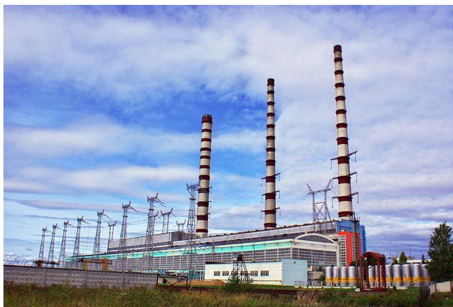
The Lukoml Thermal Power Station in Belarus. Permission Under CC BY-SA 3.0 en.wikipedia.org/wiki/File:Lukoml_power_station_20090919_02.jpg
